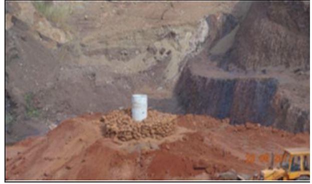
A view of the well from a distance
