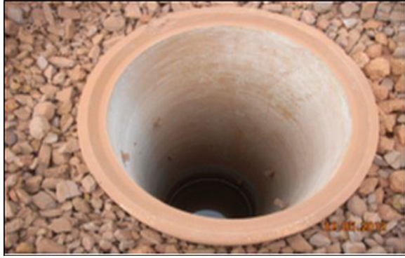
Inner view of well showing perforations
