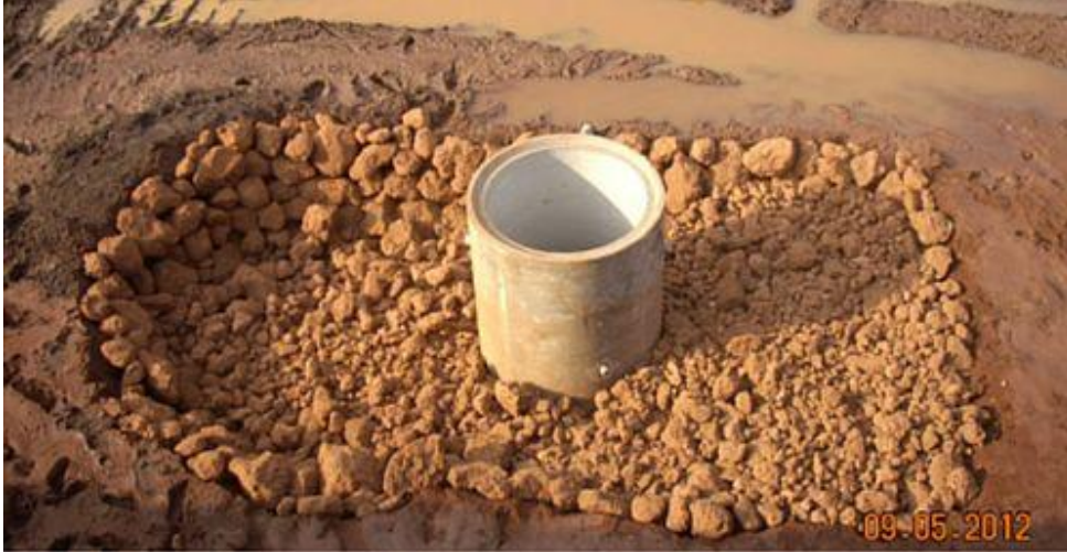
Base point of well with rubble layer around it
