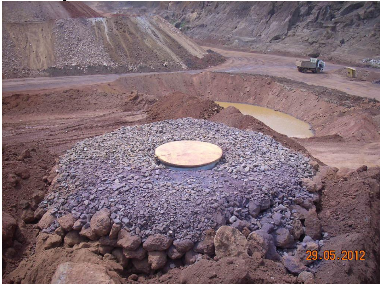
Well covered with metal cap for safety
