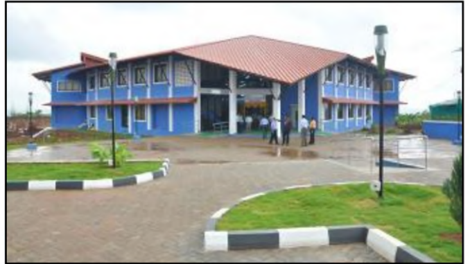
Engineering College - Mining Engineering Block
