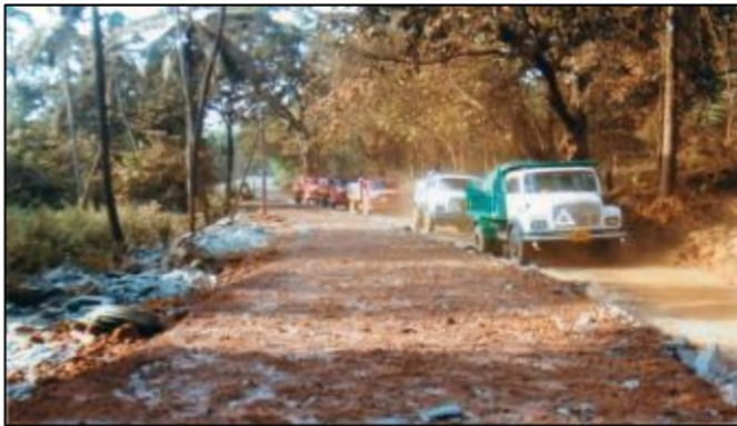
Before - Road Widening & Asphaltting
