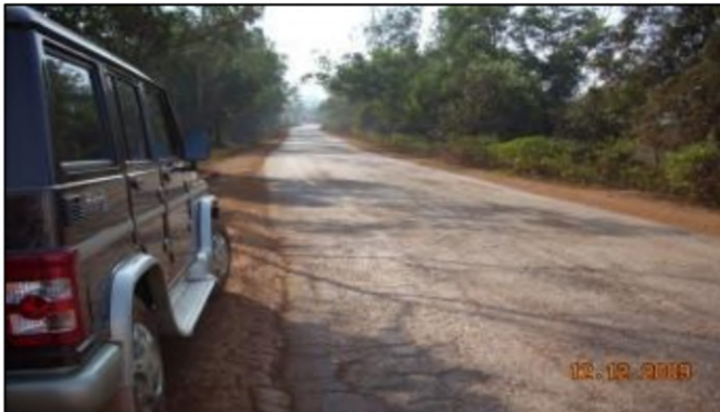
Before - Road Widening & Asphaltting
