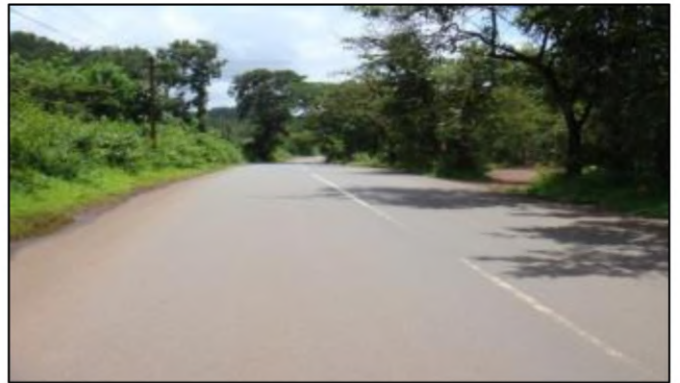
After - Road Widening & Asphaltting
