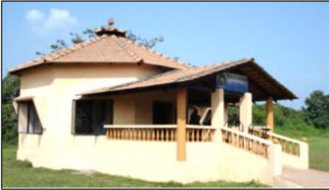
Construction of Child Friendly Anganwadi
