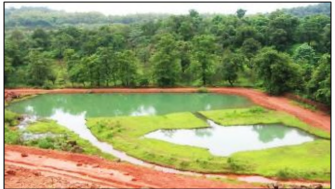
Provision of Settling Ponds Ensuring Discharge of Clear Water
