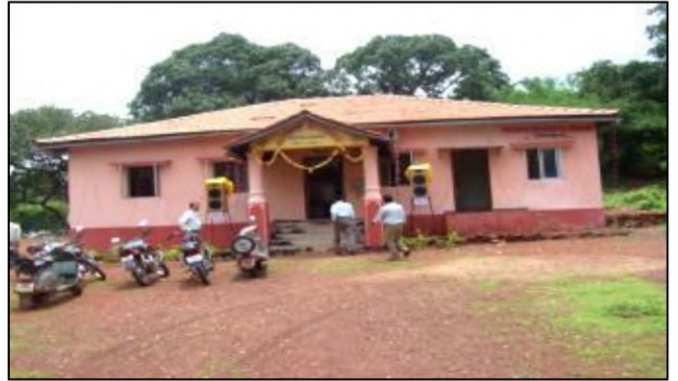
Construction of School Building
