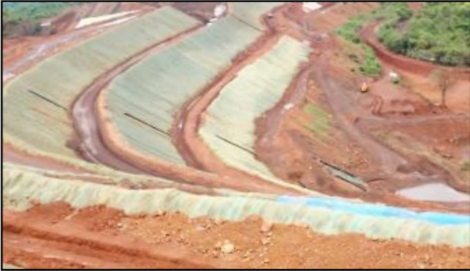
Use of Geo-textile on Dump Slopes for Slope Stabilization & Erosion Control
