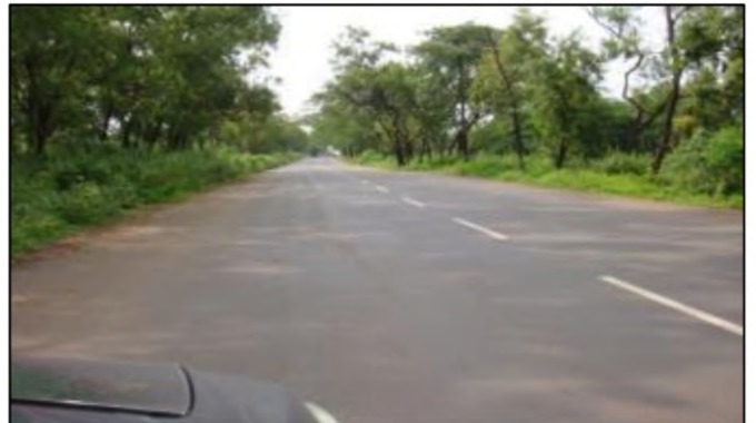
After - Road Widening & Asphaltting
